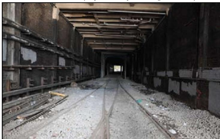
The underpass at Railway Square. The original 1855 structure is beyond the steelwork near the centre of the underpass. The double track was gauntleted following electrification of the line. Image: David Taylor
